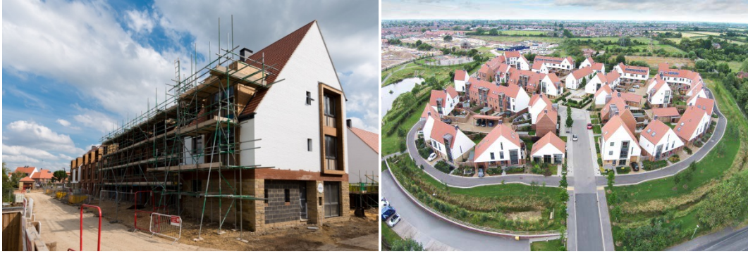
Phase 2 homes under construction, 2013
